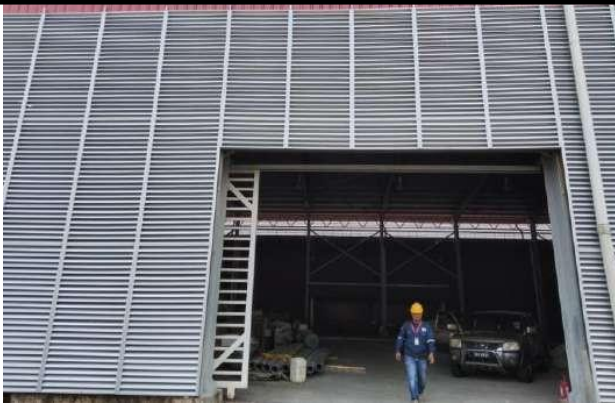
INSTALLATION OF LOUVERS AT PPMSB
