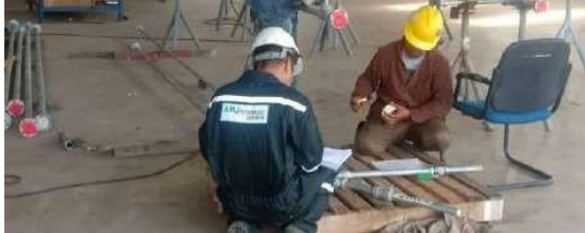
Fabrication of piping works for Exxon Mobil
