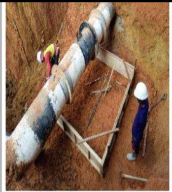
CONSTRUCTION OF VALVE CHAMBER
