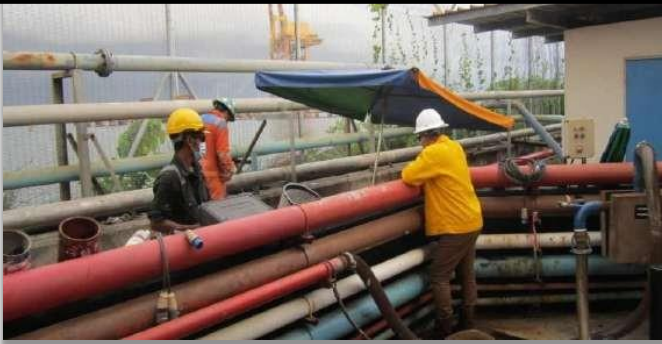
EPCC PRODUCT PIPELINE REPLACEMENT AT PENANG PORT FOR PRAI FUEL TERMINAL
