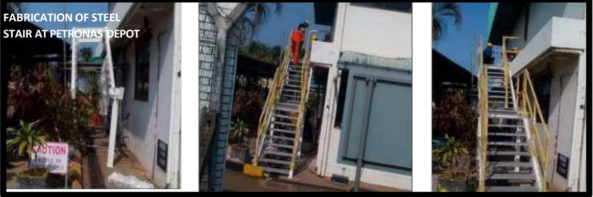
PROVISION OF UPGRADING FENCING WORKS AT JALAN WIKHAM OFF JALAN AMPANG HILIR, KUALA LUMPUR
